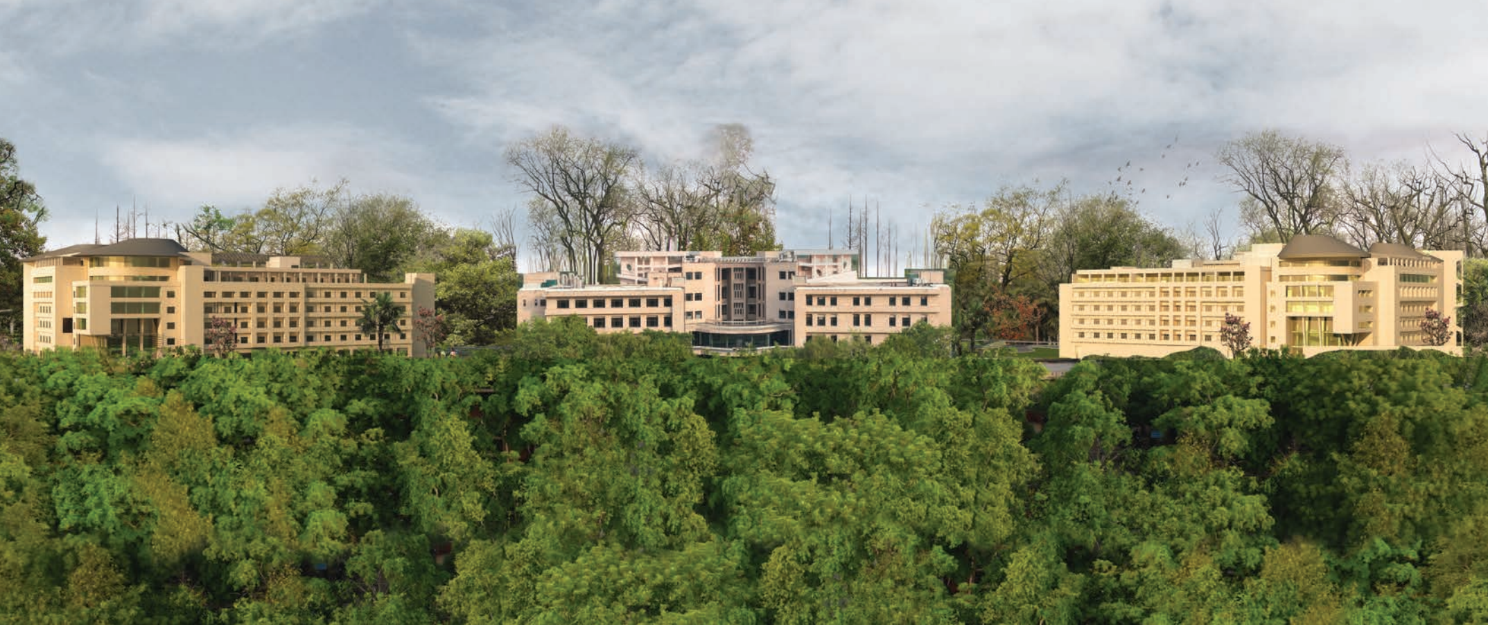
Rendered images of building 99B and 99C with photograph of LHC and foliage in the middle
